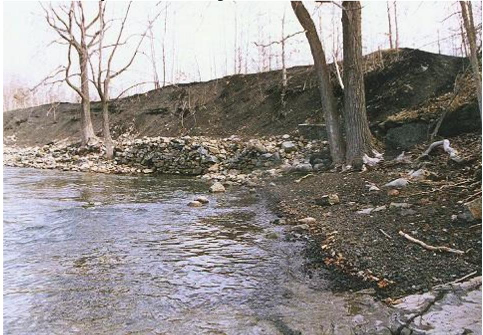
The two-tiered log cribbing structure, stretching 150 feet along the salmon pool below Willsboro falls, has been completed by Moriah Shock inmates under the supervision of John Northup, ENCON Supervisor. Work was hard and dirty due to a 35-foot tall embankment of loose black ash residue from the former pulp mill, upstream ledge rock, and downstream timbers and concrete. Nevertheless, John Northup once again illustrated his skill at turning BRASS designs into reality.
